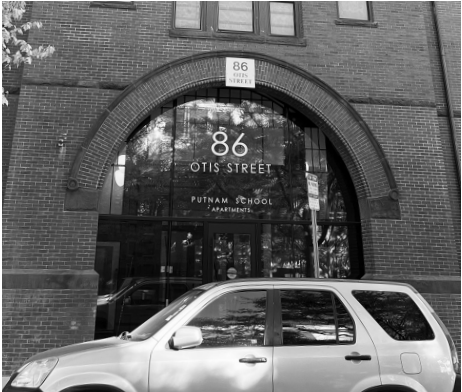
The Cambridge Housing Authority's Putnam School Apartments development at 86 Otis St., East Cambridge, seen Oct. 25.
